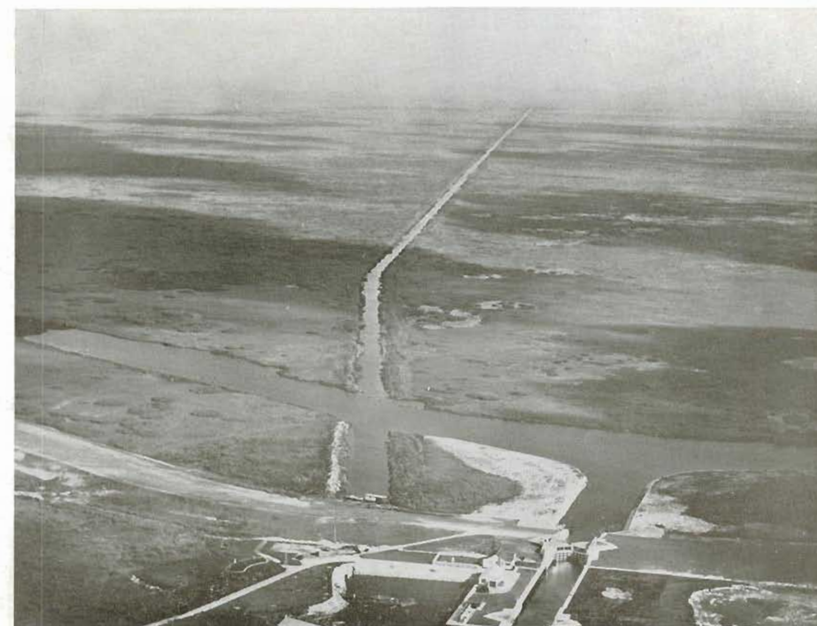
Locks Near Moorehaven in the Foreground, with West Shore Shallows of Lake Okeechobee and Dredged Channel Extending Toward the East. Dredged Channel Immediately East of Locks Leads Around Lake Rim.
