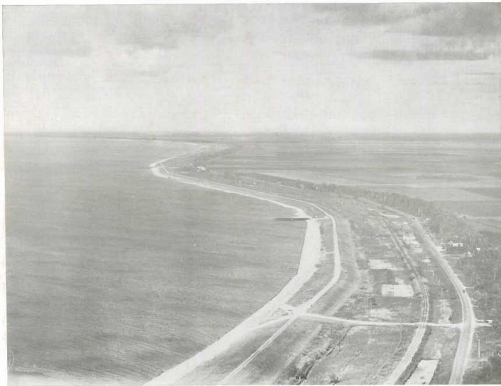
For Sixty Miles This Huge Dike, 200 Feet Wide at the Base and 34 Feet Higher Than The Lake Surface, Gives Flood Protection To Booming Everglades Cities. In Time of Threatening Storms, Massive Steel Hurricane Gates Are Shut, Making A Wall Of Defense Against The Waters.
